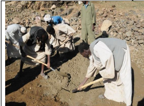
Community efforts to construct check dams and ponds
