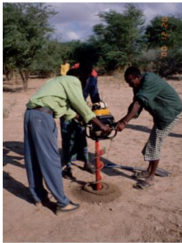
Drilling by engine auger
